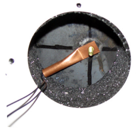
Figure 4.2.1-3: SOLAR TANK SENSOR INSTALLATION
