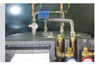
**5-8** Connect the 18" flexible stainless steel tube to the HPAK's cold inlet (left side) and the to tank's solar pump suction connection as indicated in the picture.
