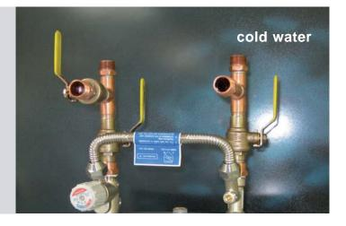
**5-7** Install the 15" stainless steel flex tube cold-water cross-over pipe.
