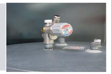
**5-3** Using Teflon thread tape, install the Honeywell cold water adaptor to the tank's top cold inlet port located on the right side of the tank.
